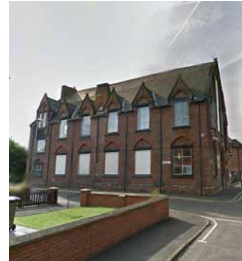
3. The Old School House, Thirsk Street
