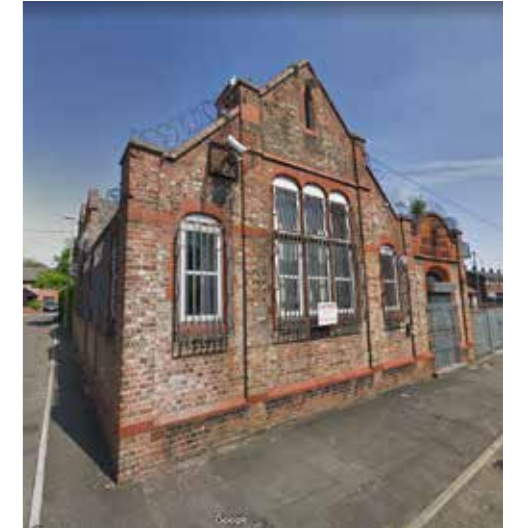
4. The Old School House, Thirsk Street
